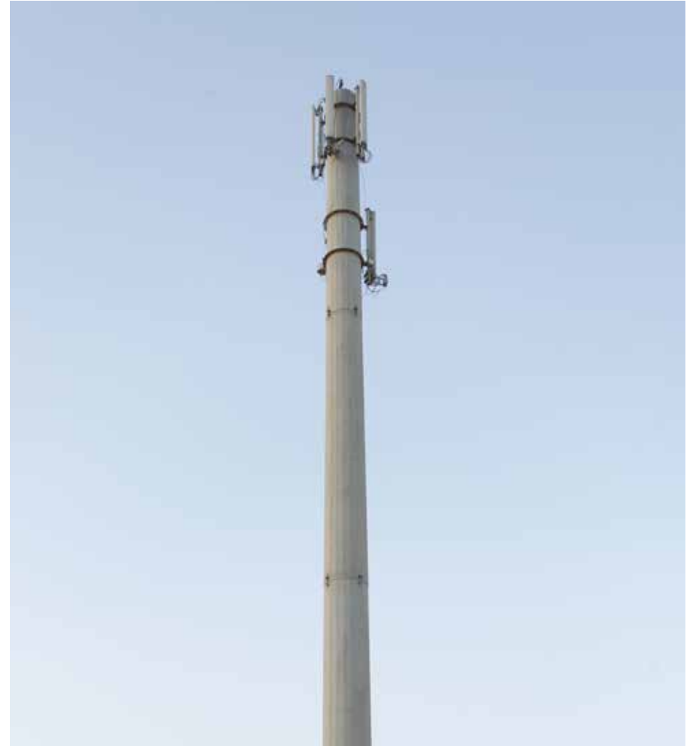
Standard monopoles are used to support antennas & dishes.
