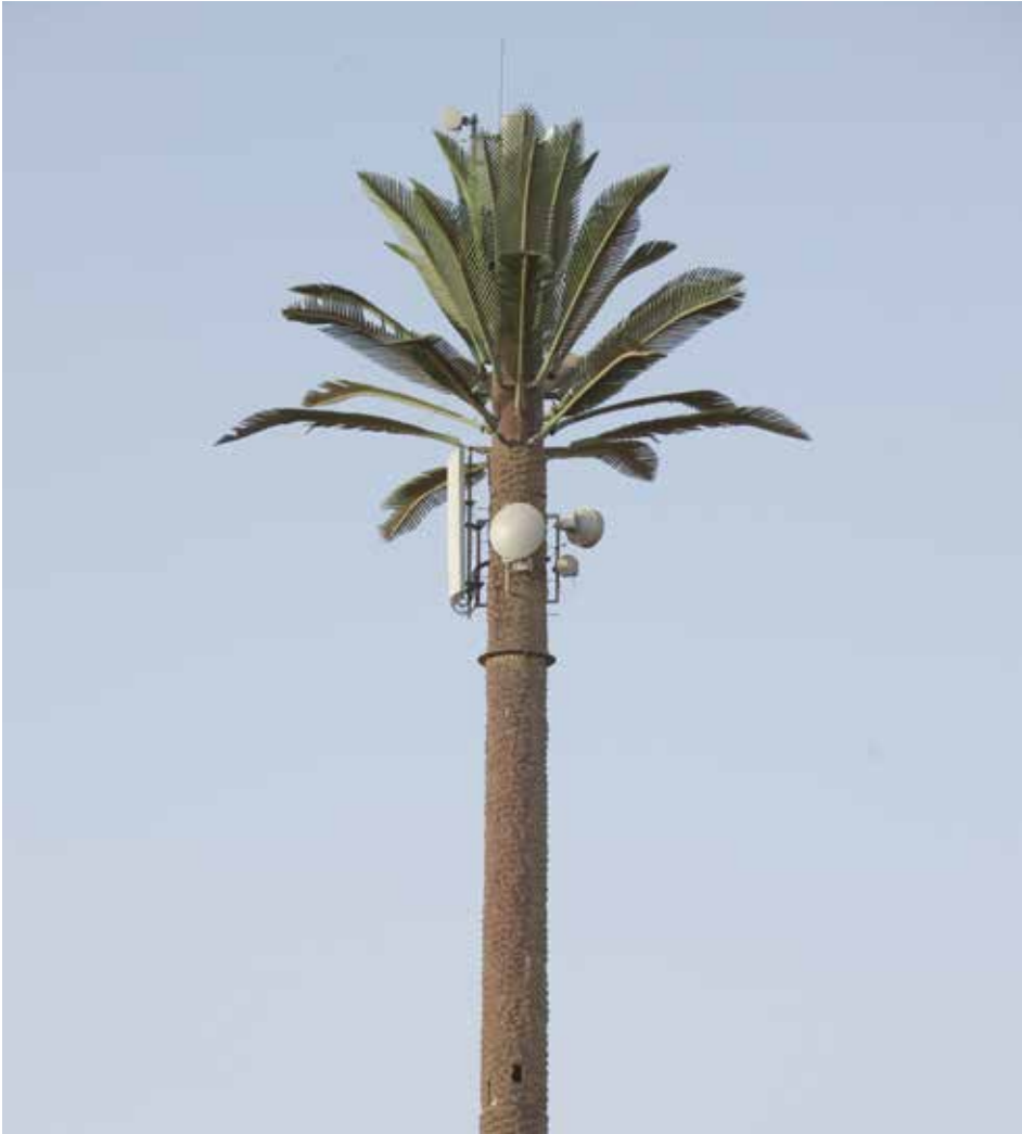
Palm trees monopoles, submitted with a camouflage & branches to hide antennas & dishes
